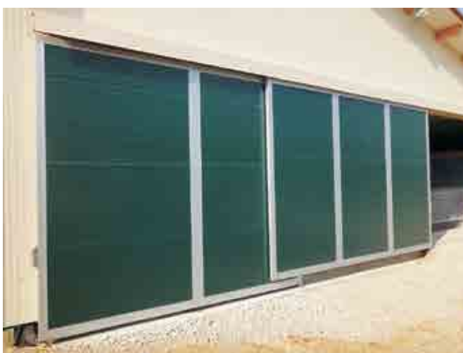
Sliding door, aluminum frame system with ISO panels, folding plates and hook lock.
