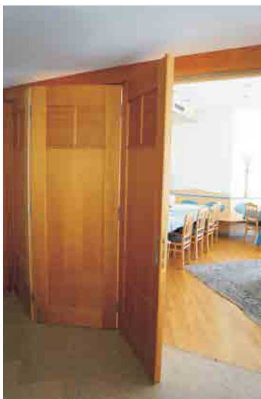
Recessed guide track eliminates the trim hazard across the threshold. Doors with flush handles.
